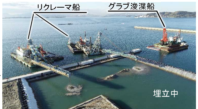
[岸壁築造工事]
