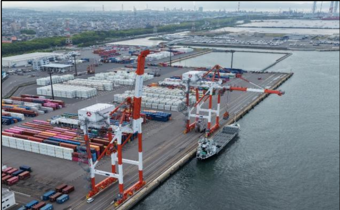
Introduction of Two Inverter-Controlled STS Cranes
